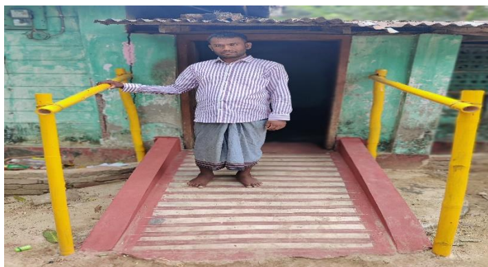
Photo: Ramp with handrail for toilet entrance
