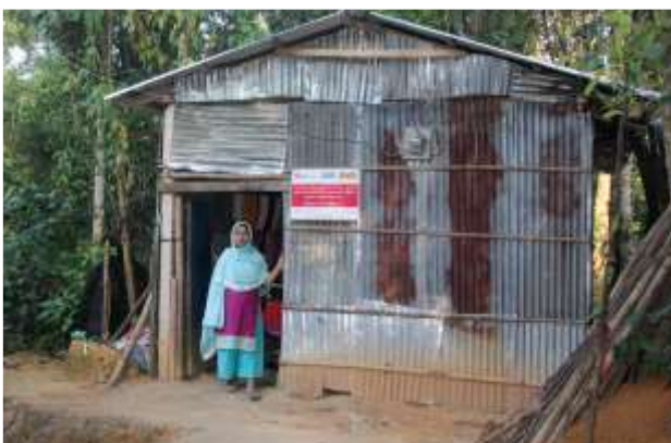
Delowara in front of her newly built simple house of two-rooms.
